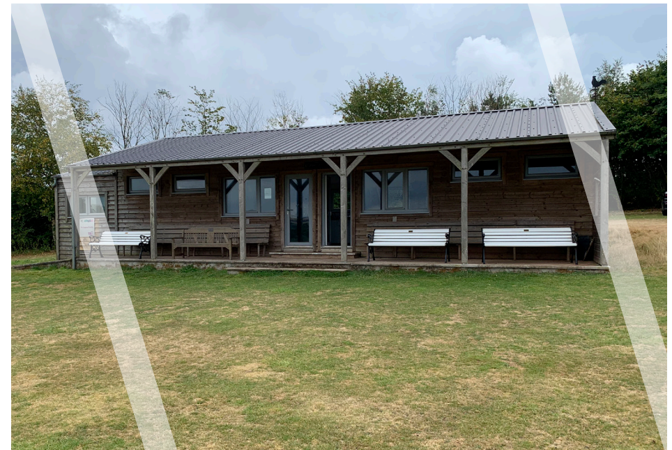
Fig 3.1.8 PV installation at rear of Harberton CC
