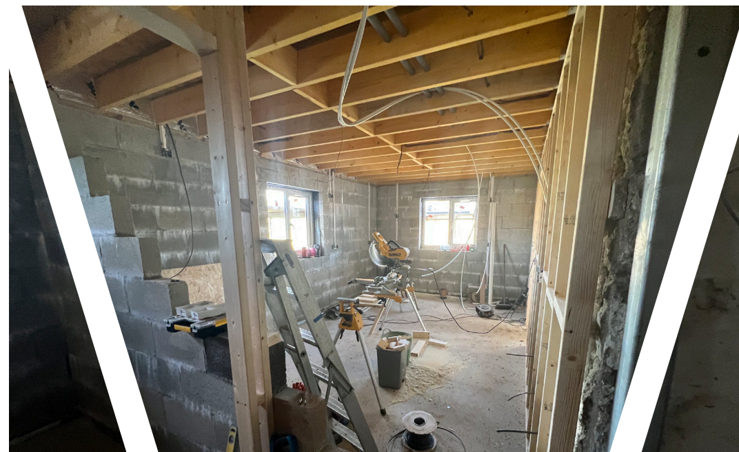
Fig 1.4 Modernisation and expansion work at Tavistock Cricket Club
