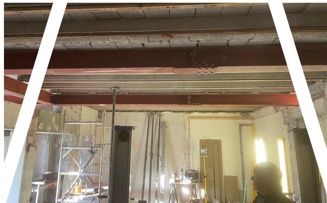
Fig 1.5 Improvements to the pavilion at Plympton Cricket Club
