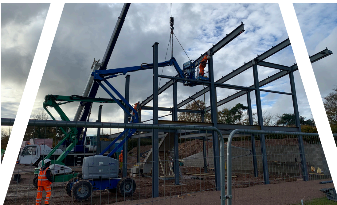
Fig 1.7 Steel erection for new pavilion at Budleigh Salterton Cricket Club
